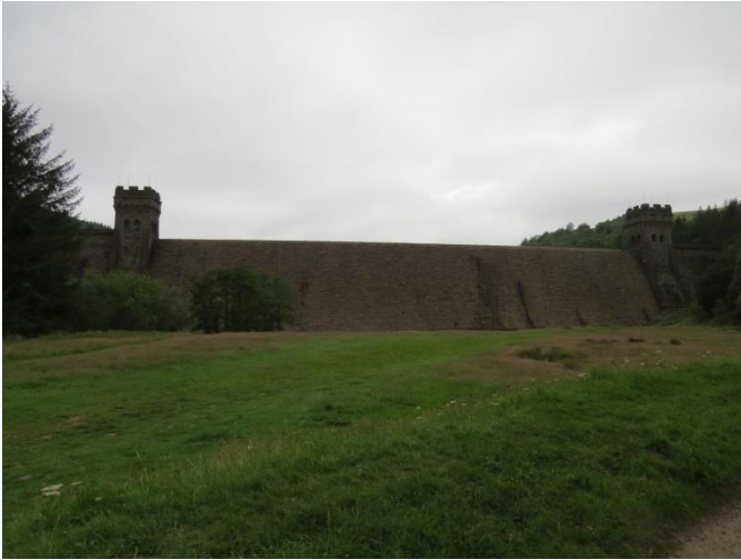
Derwent Water Dam Wall
